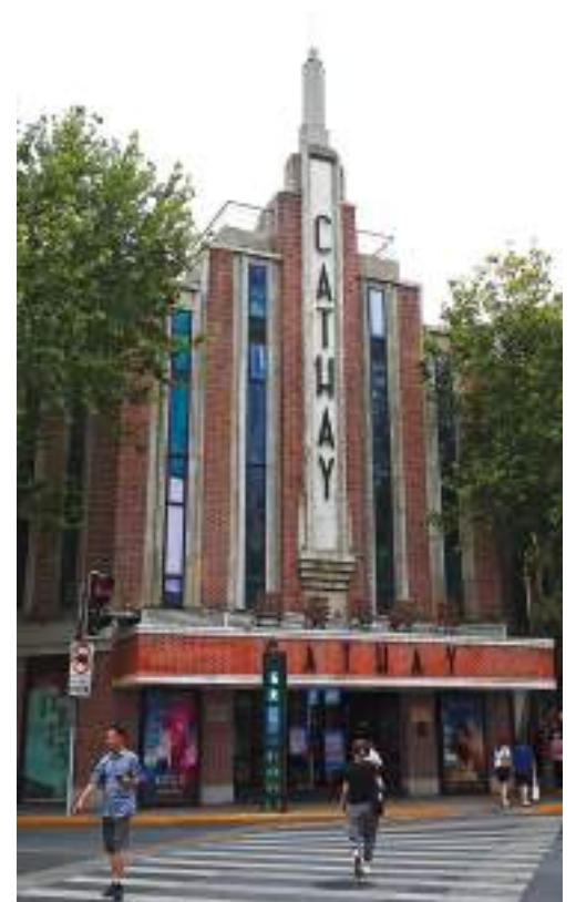
The Cathay Theatre, a time-honored cinema on Huaihai Road, suspended operations for renovations this week. — Dong Jun
