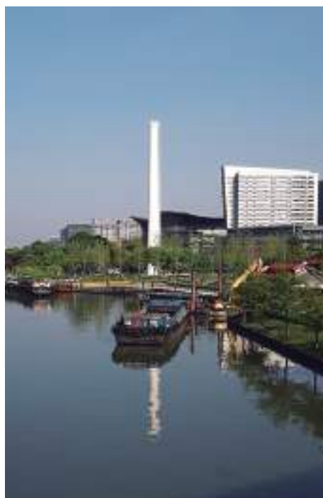
A tourist wharf is taking shape along Suzhou Creek, paving the way for the launch of cruise services next month.
