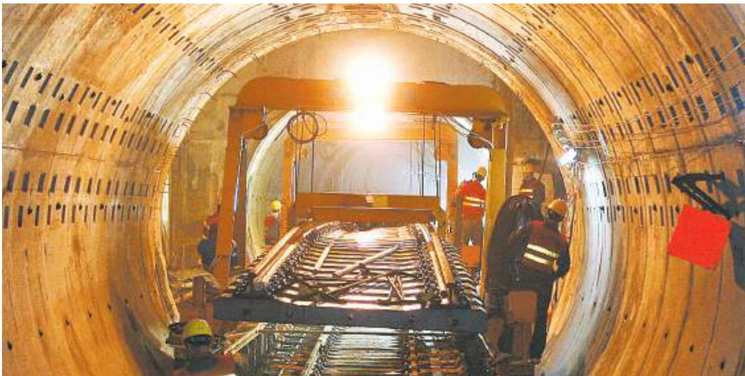
On March 1, 2012, the tunnel for Phase 1 of Metro Line 13 was linked. Since May 28, 1993, when Metro Line 1 launched its trial operation, Shanghai Metro has expanded to 831 kilometers. — Zhang Suoqing
