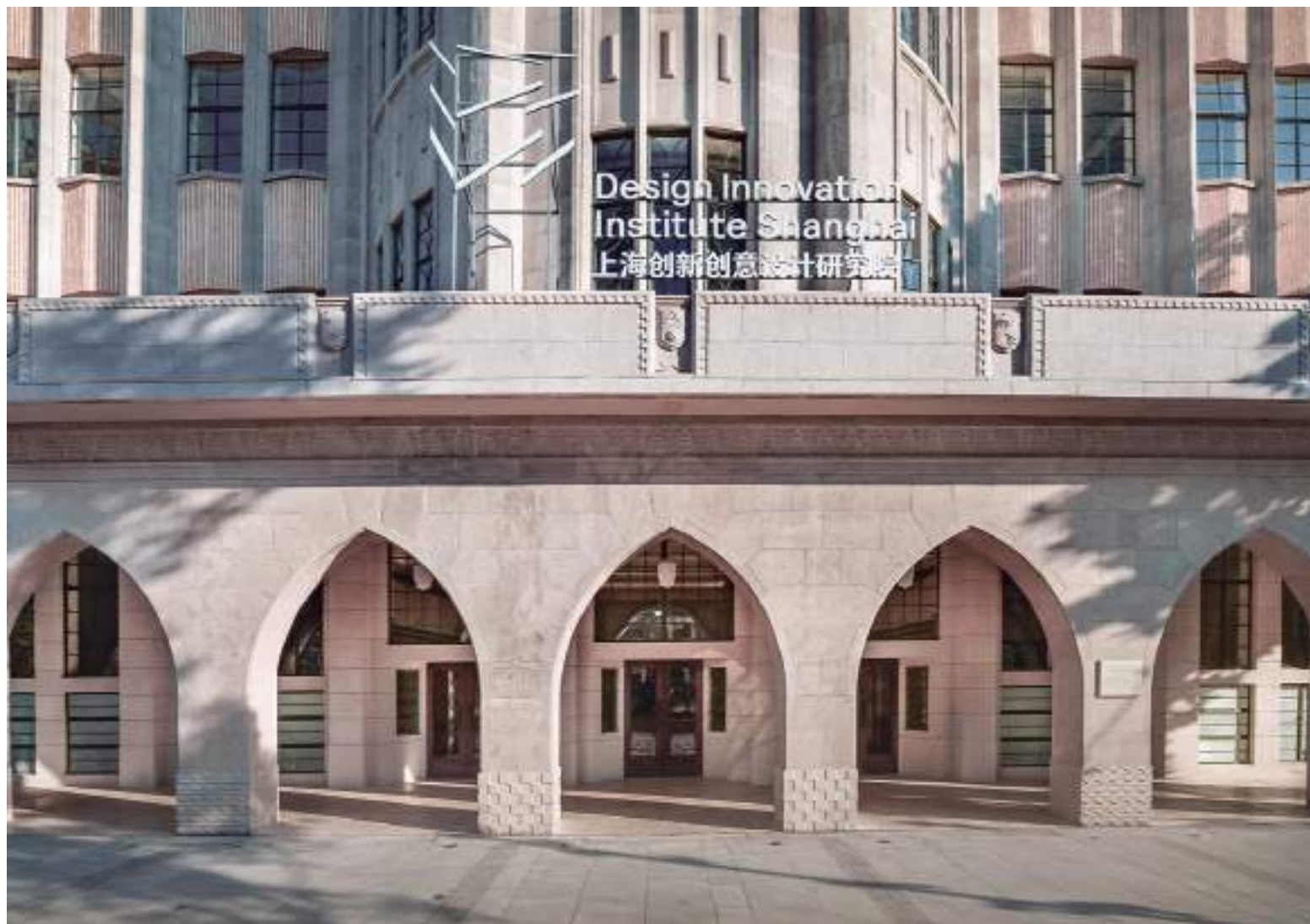
The Design Innovation Institute Shanghai is located in the North Bund central business district of Hongkou District. — Photos by Ti Gong
