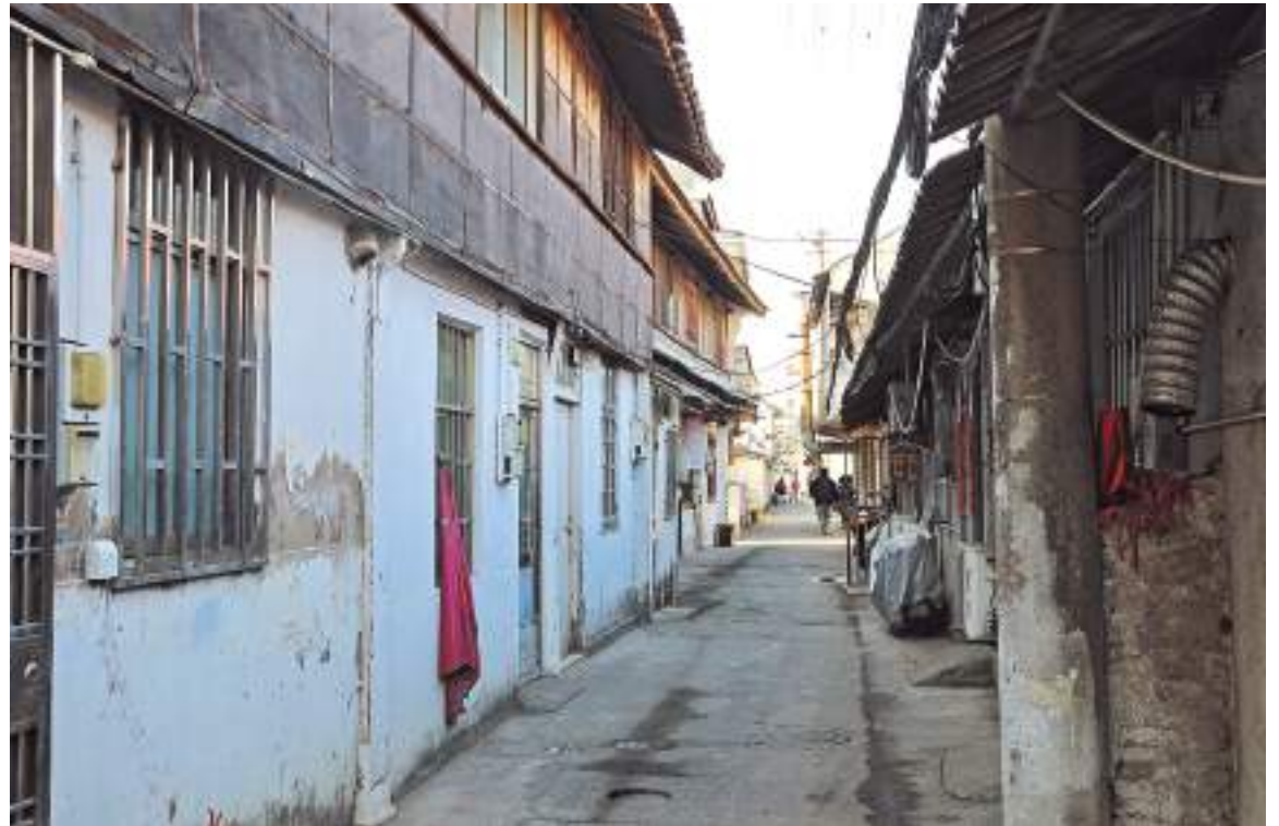
An urban village in Shanghai's Pudong New Area slated for renovation. — Ti Gong
