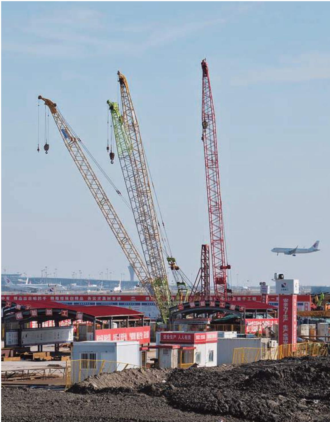
A view of the under-construction Shanghai East Railway Station. — CFP
