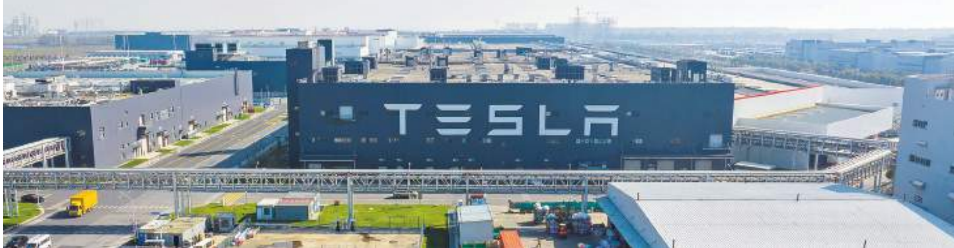
A view of the Tesla's Gigafactory Shanghai. — CFP
